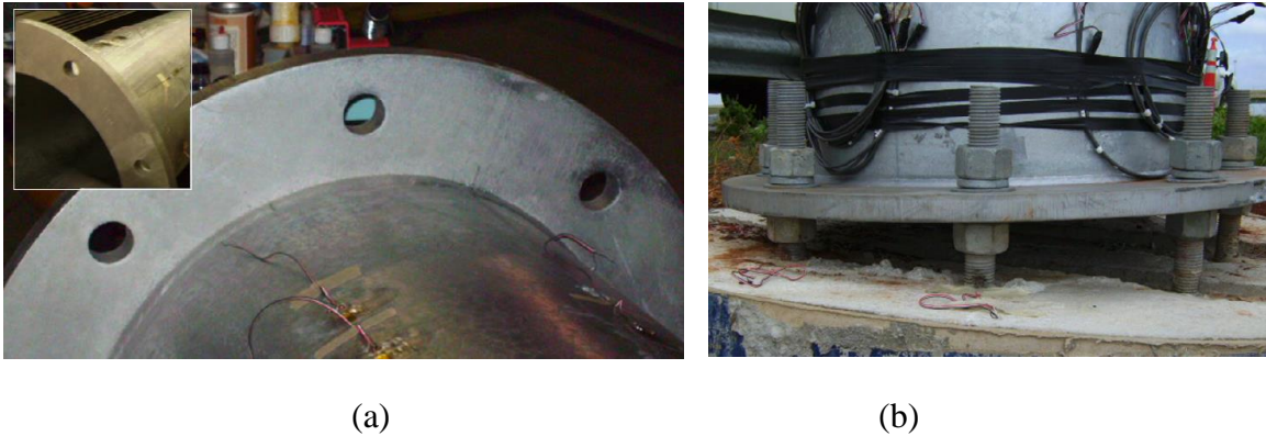
Figure 2.17 (a) Fillet-welded tube-to-transverse plate connection and (b) anchor bolt connection
