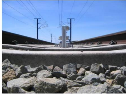
a) Ballast profile lowered on the Rome-Naples HSR
