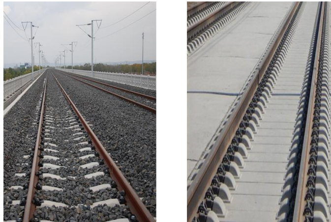
Figure 1.1 Ballasted track and non-ballasted track
