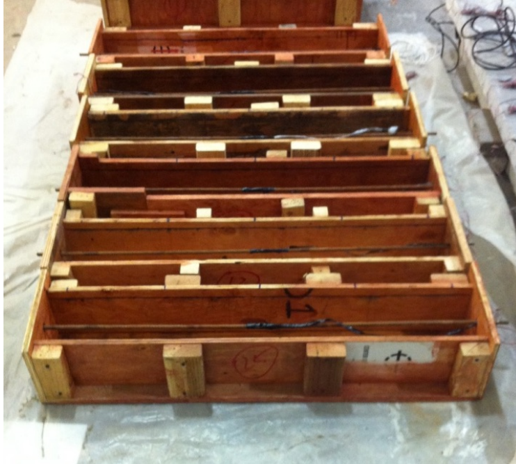
Figure 3. 9 Beam Molds with Main Reinforcement Rebar Placed
