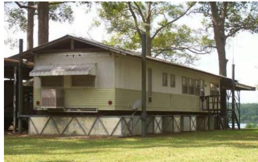
Figure 30. A floating home with EPS base in rural Louisiana. EPS blocks are encased in a steel frame (E. English)
