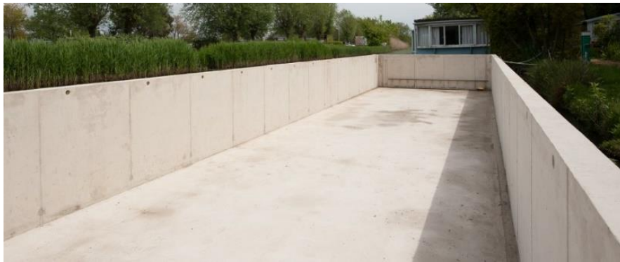
Figure 44. Hollow reinforced concrete floating base. (Floating Homes Ltd)
