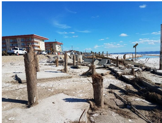
Figure 2. Home ripped off foundation due to Hurricane Michael storm surge in Mexico Beach, Florida
