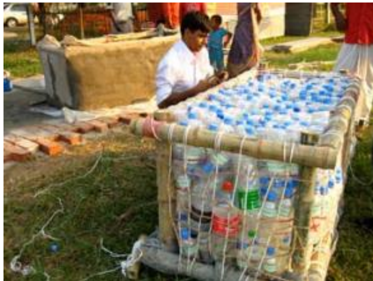
Figure 39. Recycled plastic bottles encased in bamboo use as a buoyant base for the LIFT house (E. English)
