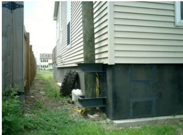
Figure 35. The buoyant steel base is attached to wooden guide posts on its exterior (E. English)
