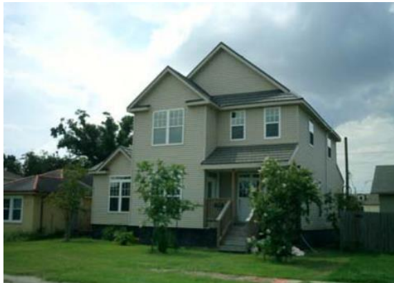
Figure 34. New Orleans floating home which sits in a hollow steel box (E. English)
