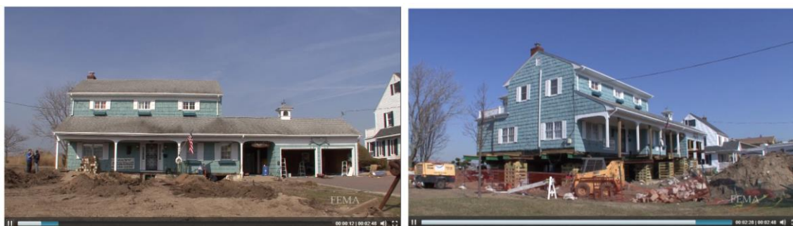
Figures 3.4 & 3.5: FEMA, Freeport, Long Island house before and after elevation, Homeowner elevates Historic House, https://www.fema.gov/media-library/assets/videos/82505 , (accessed July 2, 2018).
