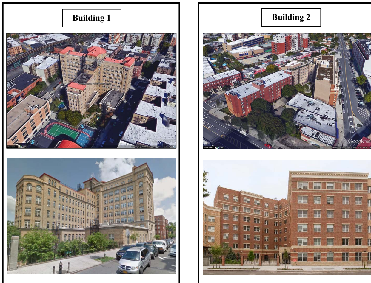
Figure 1. Field study sites. a) Building 1 and b) Building 2 (Photo credits: Google Maps and WHEDco: Women's Housing and Economic Development Corporation; Bronx, NY).
