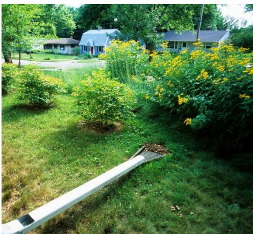
Figure 3.11: Example of a downspout extended to a rain garden
