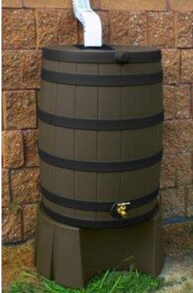
Figure 3.12: Downspout diverted to a rain barrel
