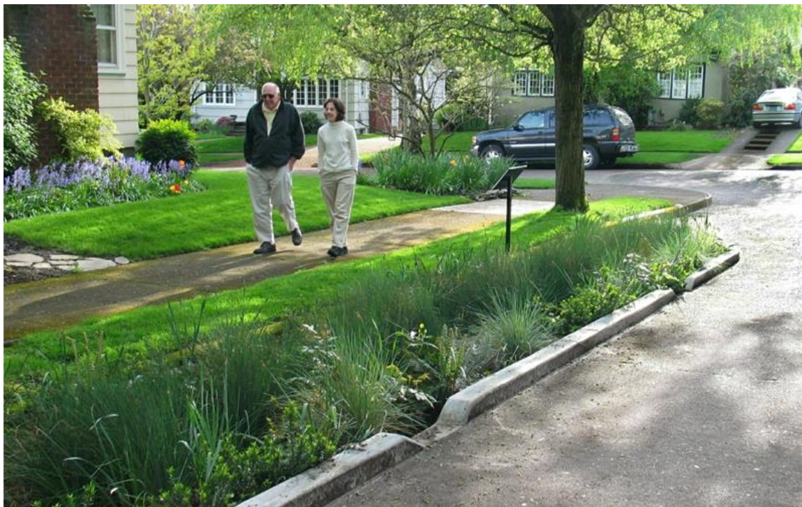
Figure 3.21: A bioswale in a residential neighborhood in Portland, Oregon.
