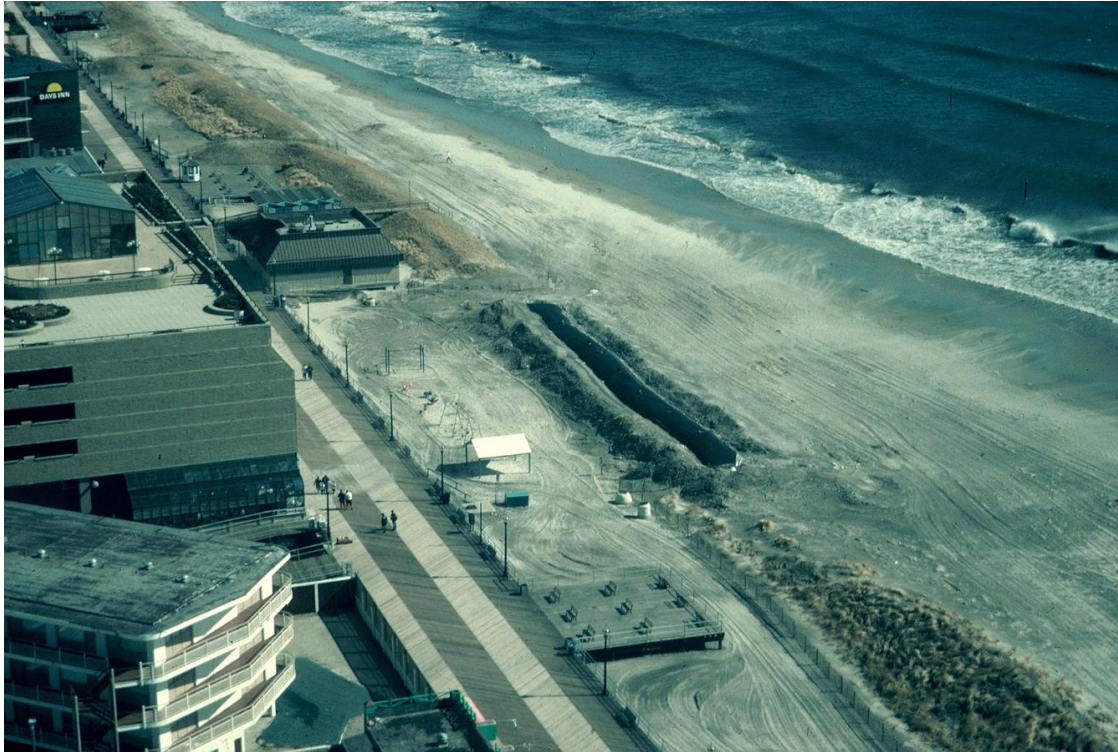
Figure 16: Geotubes in practice. Geotube being emplaced on shoreline prior to being buried with sand (Nordstrom, 2019).
