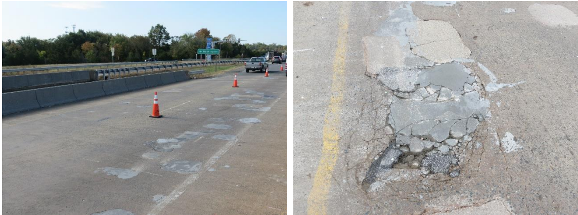
Figure 2-1. Deck deterioration.
