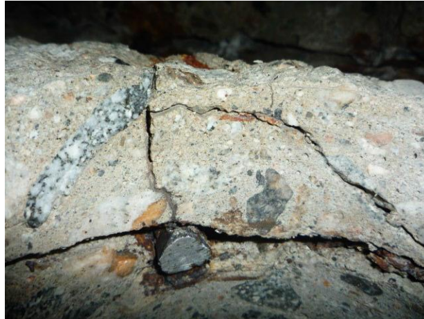
Figure 2-2. Extensive cracks caused by the corrosion of reinforcing steel.
