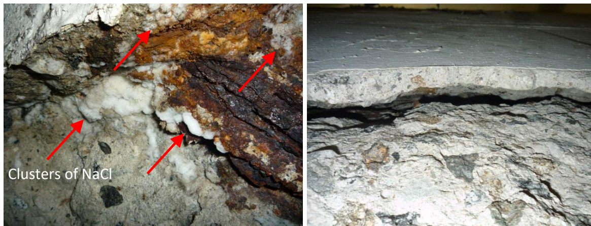
Figure 2-4. Delamination caused by corrosion.
