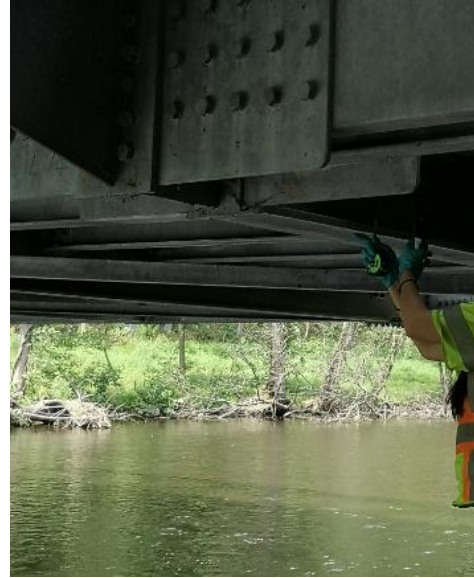
(b) Inspection of the Floorbeam
