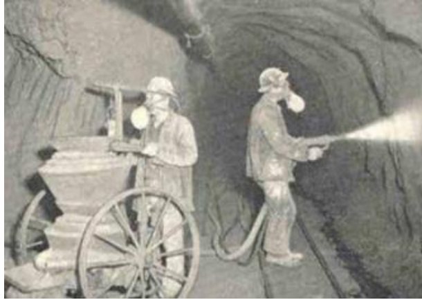
Figure 2.2 – Lining a tunnel with guniting using a double-chamber gun during the 1920s (Morgan and Bernard 2017)
