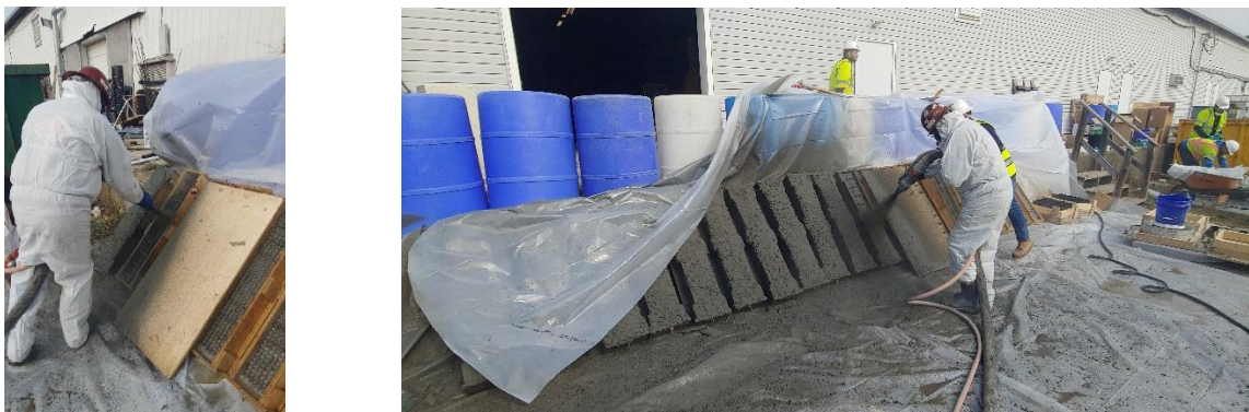
Figure 3.14 – Shotcrete laminate casting
