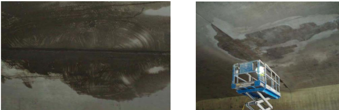
Figure 2.11 – Repairs on underside joint of roof of a tunnel bridge (Wenzlick 2007)
