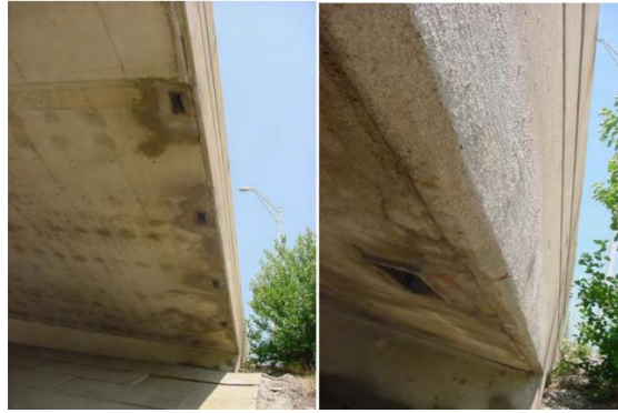
Figure 2.10 – Br. A2175, shotcrete patches around drains now 8 years old (Wenzlick 2007)
