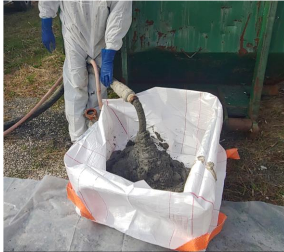
Figure 3.4 – Shotcrete run through the line
