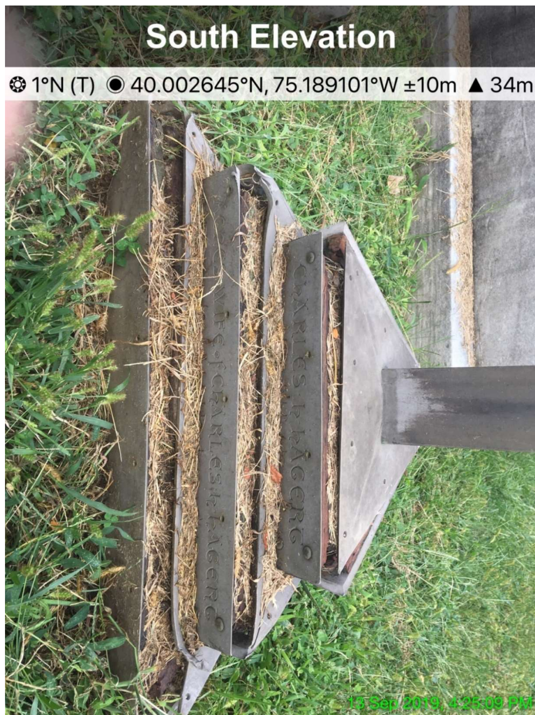
Figure 7. Solocator GPS Image. Spalling damage on metal grave marker.
