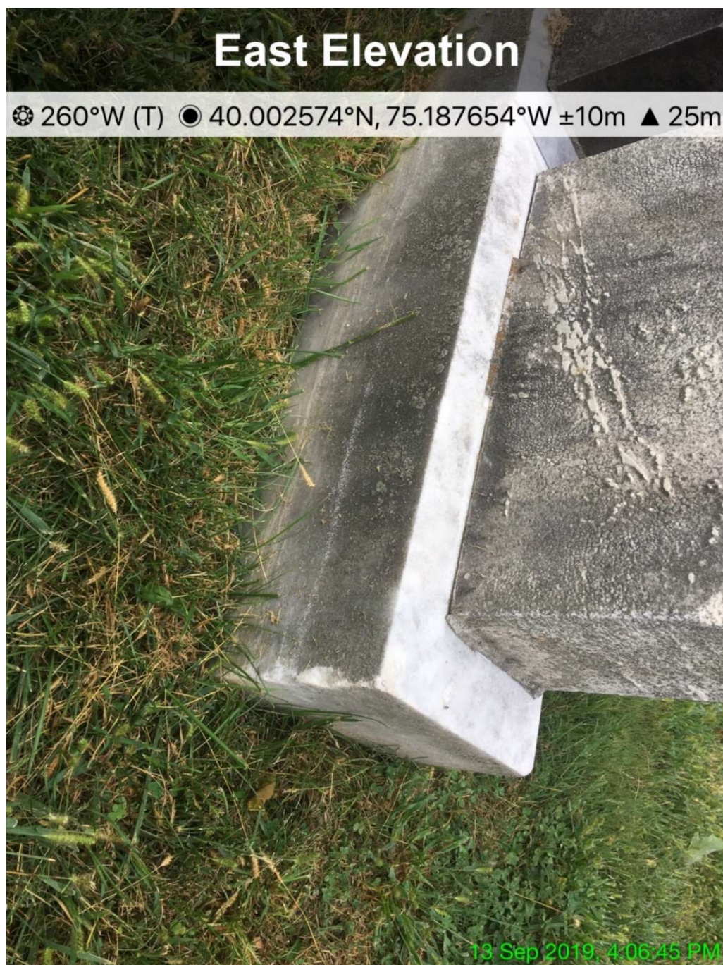
Figure 6. Solocator GPS Image. String trimmer damage may be seen in the corner and alongside the horizontal base of the marble grave marker. Photograph by Author.
