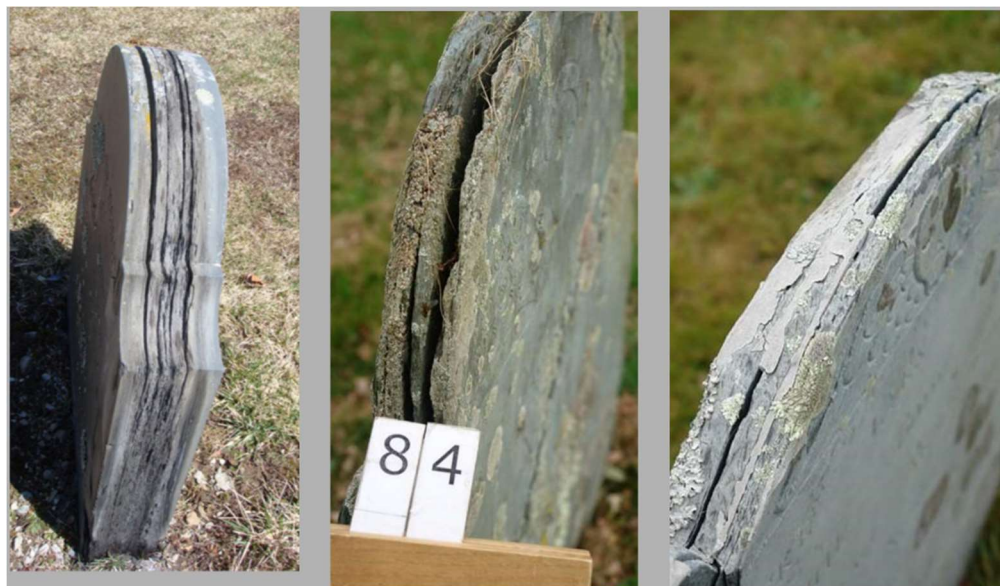
Figure 4. Slate is highly prone to chipping and flaking. Photographs by Irving Slavid in Jason Church, U.S. Department of the Interior, National Park Service, “The Challenges of Treating Delaminating Slate Headstones: New Treatments with New Materials,” National Center for Preservation of Technology and Training, posted December 10, 2014, accessed November 11, 2019, https://www.ncptt.nps.gov/blog/the-challenges-of-treating-delaminating-slate-headstones-new-treatments-with-new-materials/
