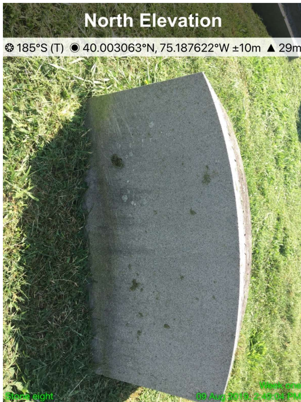
Figure 5. Solocator GPS Image. String trimmer scratches may be seen on the edge and grass stains indicating newer impact are alongside the horizontal base of the granite grave marker. Photograph by Author.
