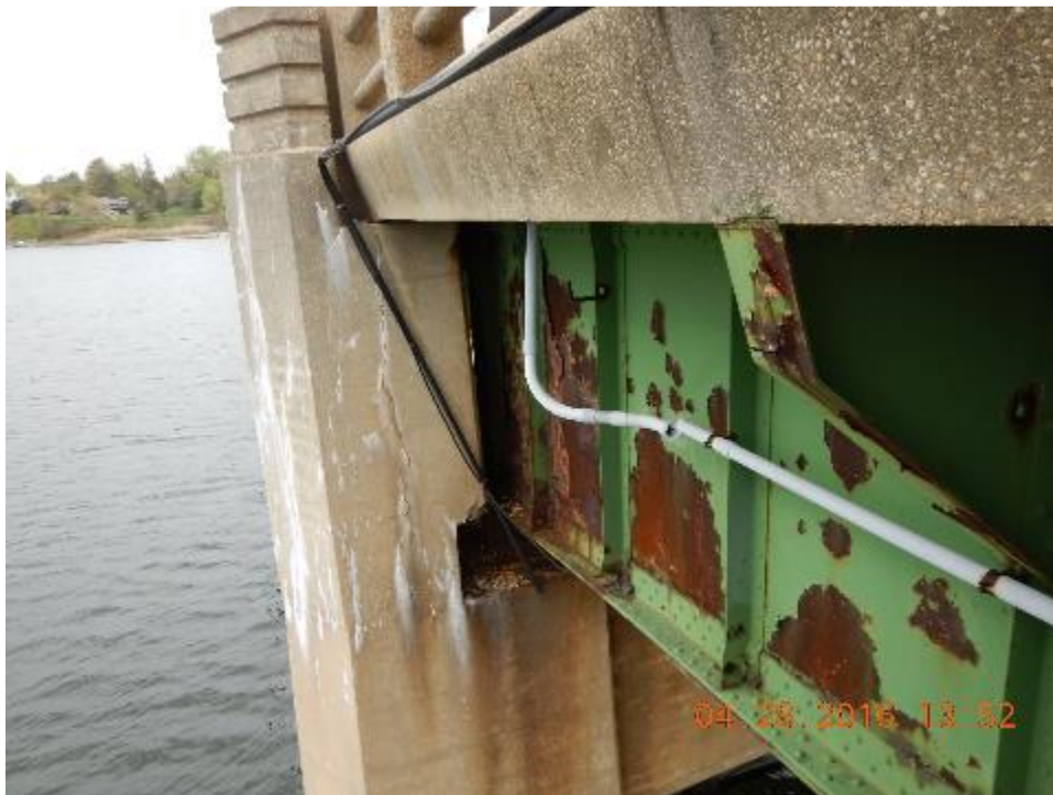
Figure C.6 - Fascia Girder at Bascule Pier (Looking North)
