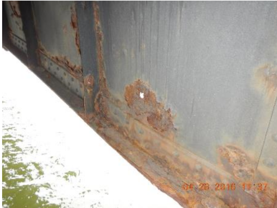
Figure C.9 - Fascia Girder (Interior View) Corrosion on Bottom Flange
