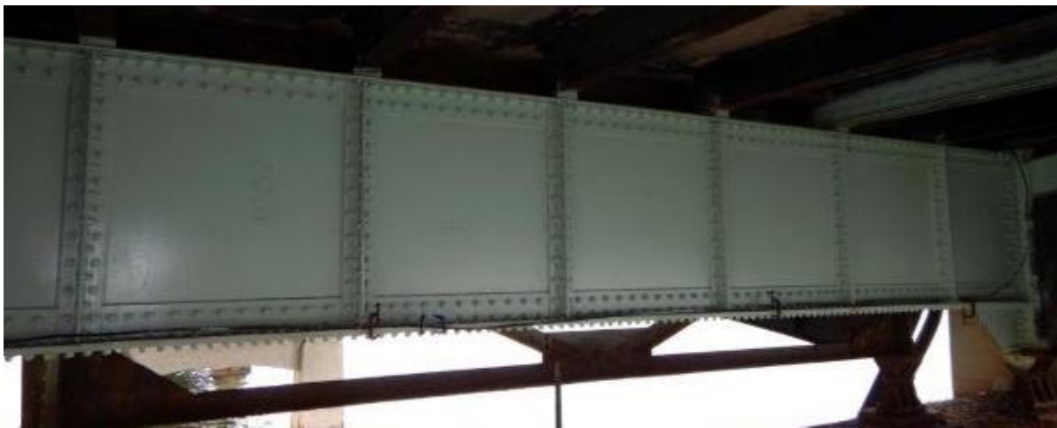
Figure 2.8 – Span 28 (Looking Northeast) Floor Beam 2016 Condition
