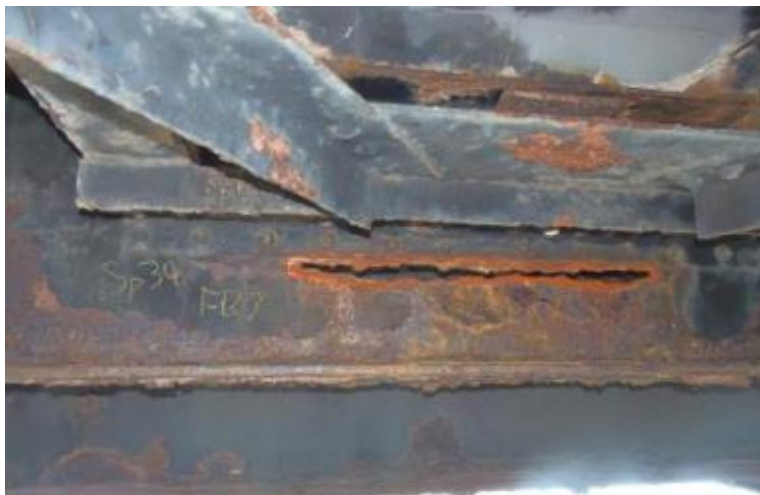
Figure 5.4 - Span 34 Floor beam 7 Section Loss along the Top Flange
