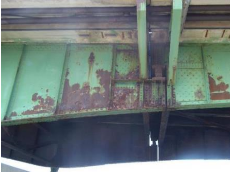
Figure 5.5 - Section Loss and Corrosion at Rocker Bearing Connection
