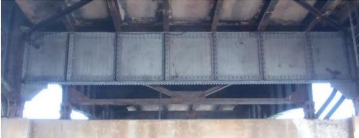
Figure 4.5 - Floor Beam following 2015 Rehabilitation
