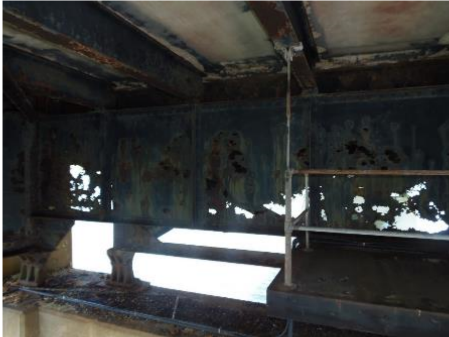
Figure C.3 - 2013 Deteriorated Floorbeam (Looking North)
