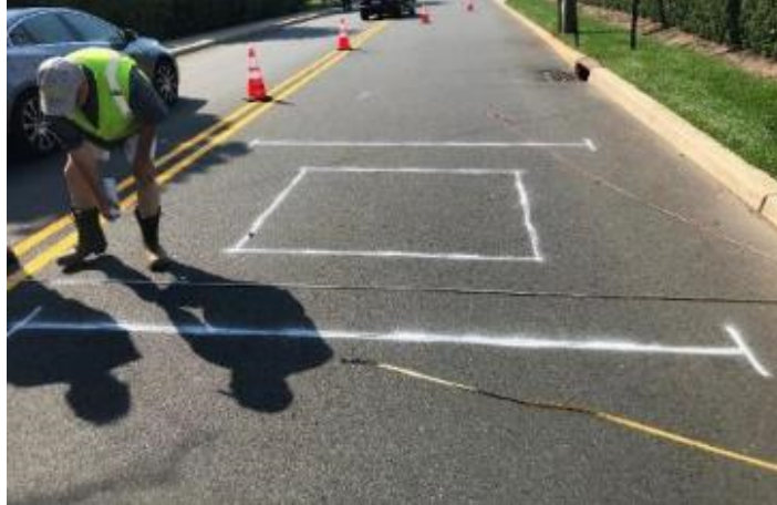
Figure 4.23 - WIM Installation Step 2
