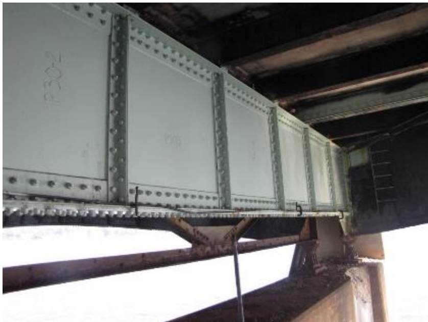
Figure C.4 - 2015 Repaired Floorbeam (Looking East)
