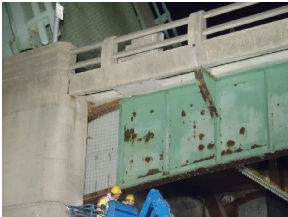
Figure C.10 - Fascia Girder Repair at Bascule Pier during 2015 Rehabilitation
