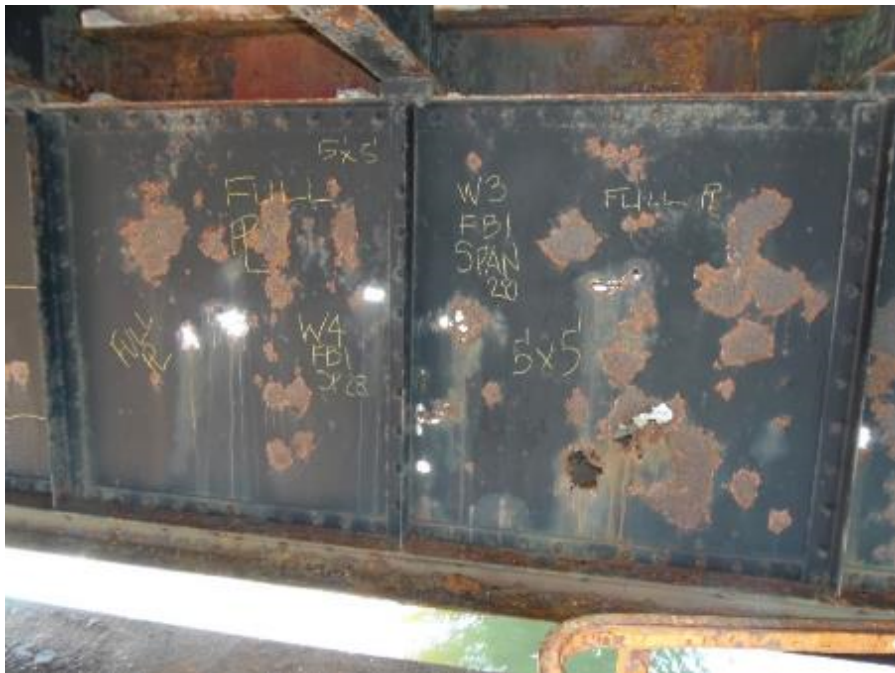
Figure C.2 - 2013 Deteriorated Floorbeam (Panels 2 and 3)
