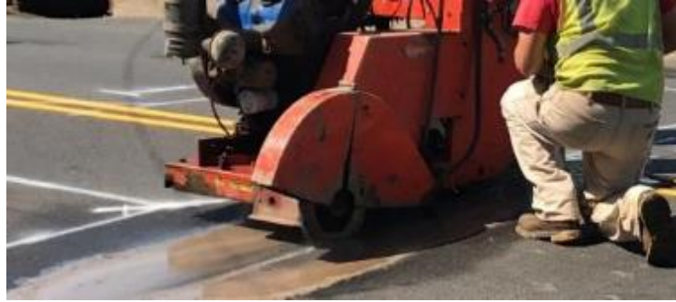
Figure 4.26 - WIM Installation Step 3 WIM saw cutting
