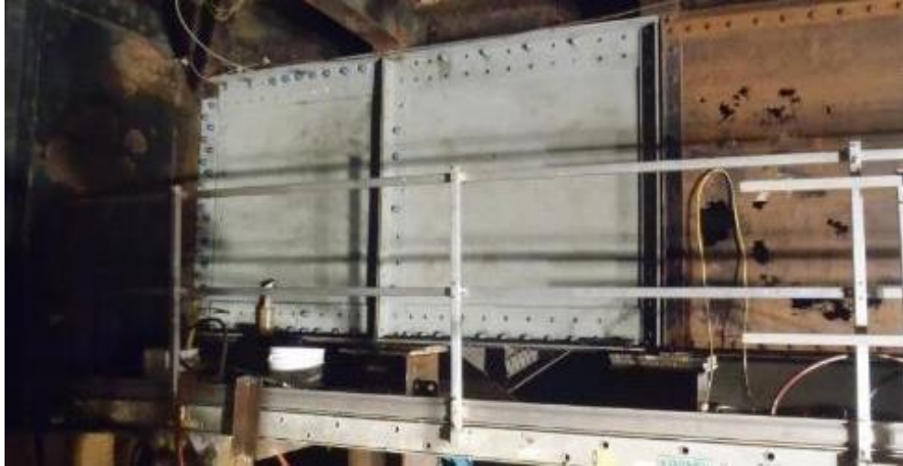
Figure 2.7 - Floor Beam at Anchor Span Mid-Repair
