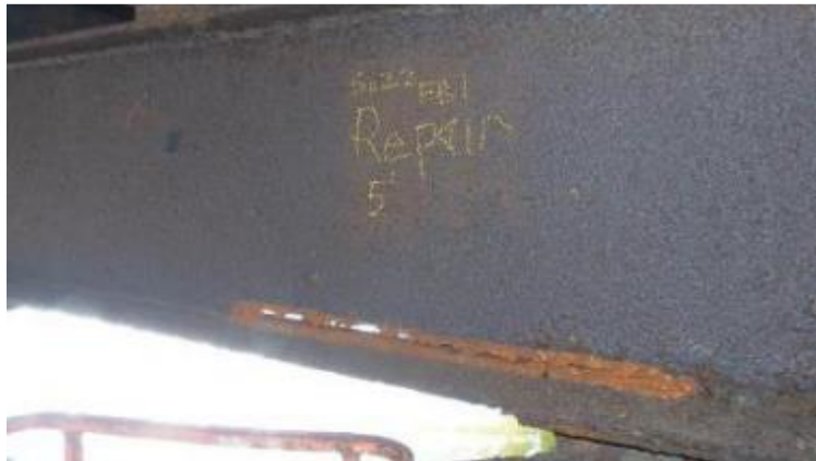
Figure 5.3 - Span 22 Floor beam 1 - 5 LF of Section Loss along Bottom Flange
