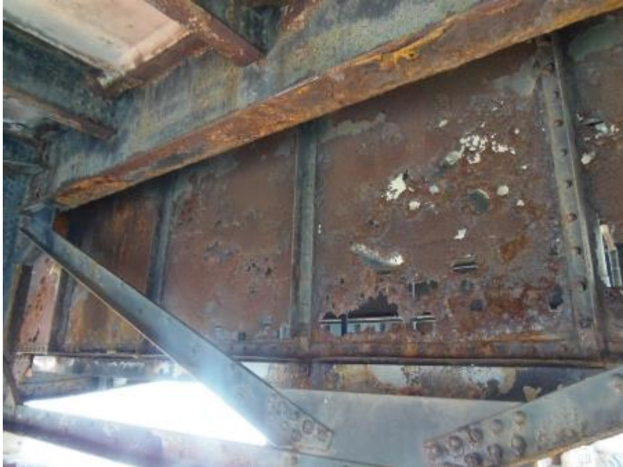
Figure C.1 - 2013 Deteriorated Floorbeam (Center Panels)
