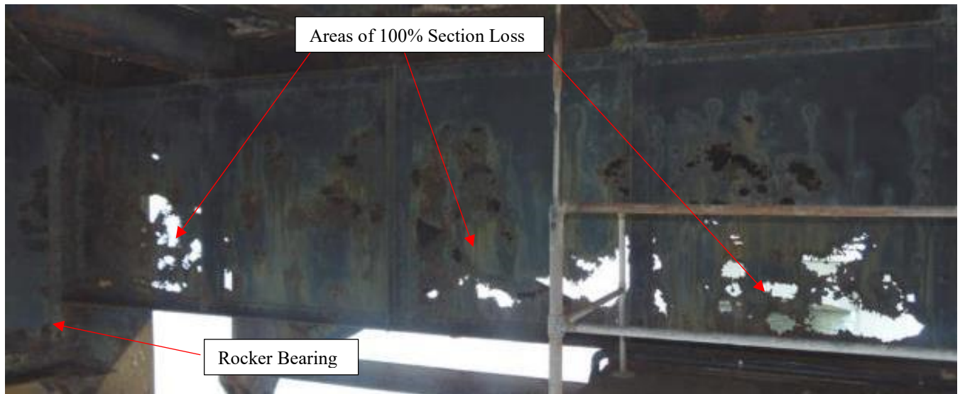
Figure 2.6 - Span 28 (Looking Northwest) Floor Beam 2013 Condition
