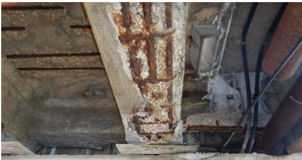
Figure 5.2 - Spalling of Concrete Deck and T-Beams (Approach Spans)
