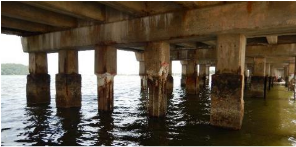
Figure 5.1 - Spalling of Pile Bents (Approach Spans)
