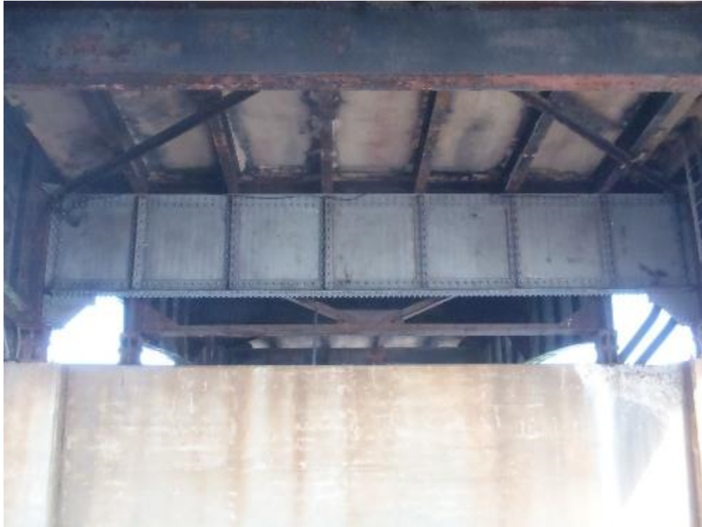
Figure C.5 - Repaired Floorbeam (Looking North)
