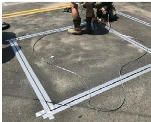
Figure 4.27 - WIM Installation of Sensors
