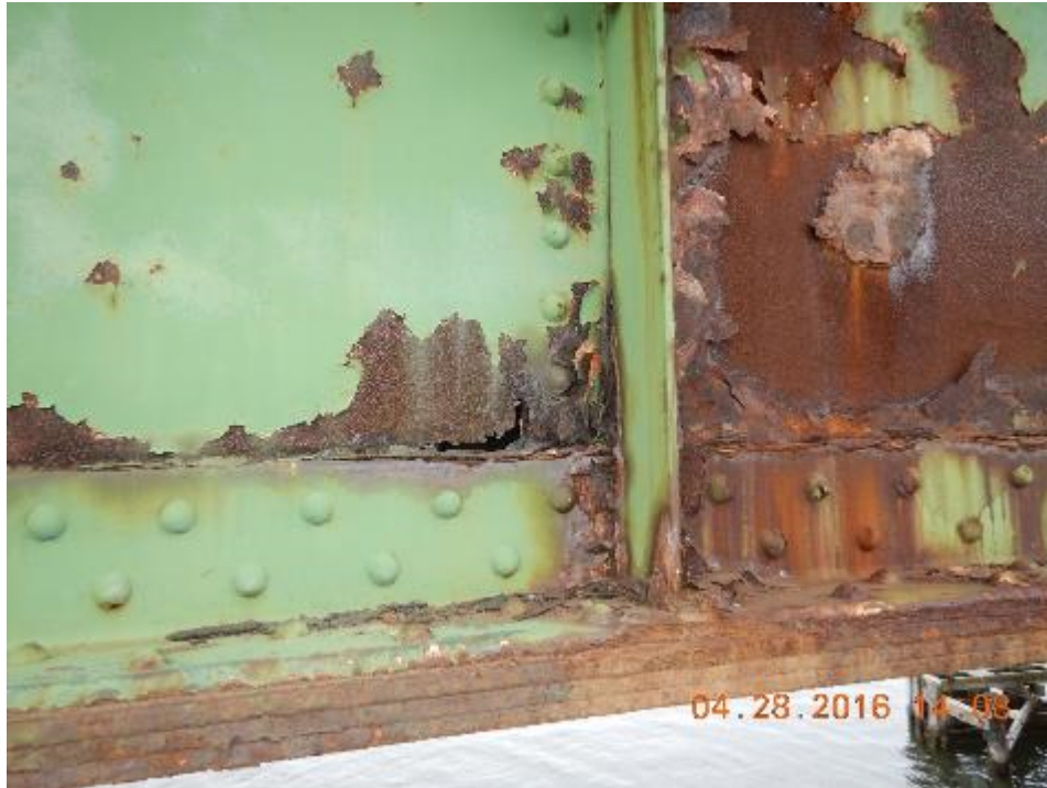
Figure C.7 - Fascia Girder Midspan Corrosion (Looking East)
