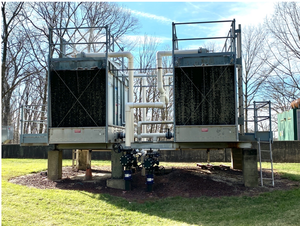
Figure 18. A two-cell crossflow cooling tower
