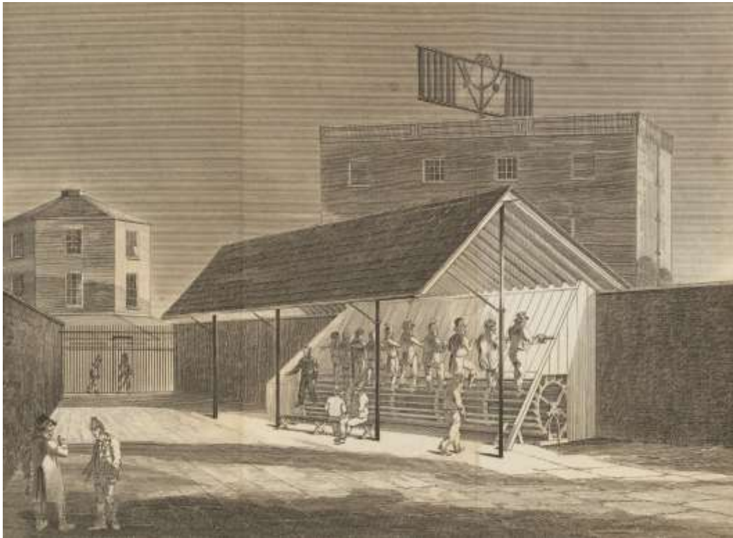
Figure 6: The treadmill at Brixton Prison. Note the weighted air-resistance fan above the prison building. Society for the Improvement of Prison Discipline and for the Reformation of Juvenile Offenders, Description of the tread mill for the employment of prisoners (London : Longman, Hurst Rees, Orme and Brown, 1823) [Courtesy of Harvard University Library]
